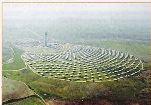
figure 16. Heliostats surround part of the central power tower at Planta Solar 10 in Spain (used with permission from Solucar Energia/Abengoa).
